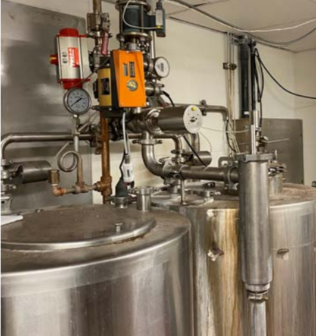
CIP upgrades at the Bridgeton, Missouri site
