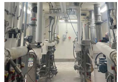
Insulation upgrades at the Slate Hill, New York site
