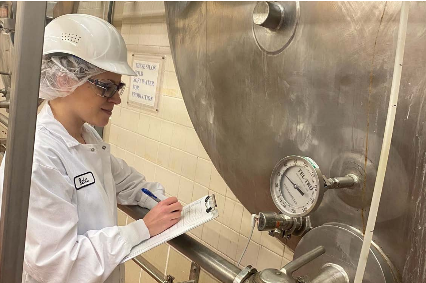
Water level sensor upgrades at the Marshfield, Wisconsin site
